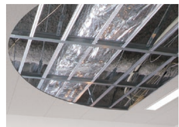
Our own anti-seismic ceiling construction technique
