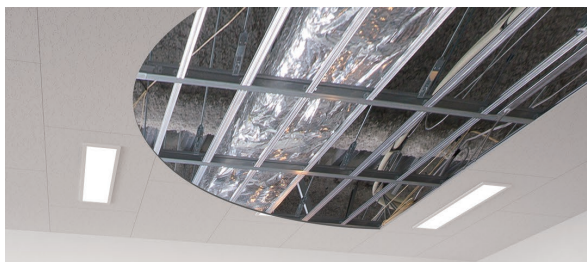
Our own anti-seismic ceiling construction technique
