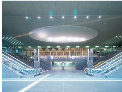
Kyoto Station Building (Kyoto)
