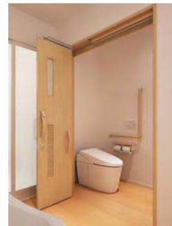
A sliding door with sufficient width to allow for easy access by wheelchair and care workers.
