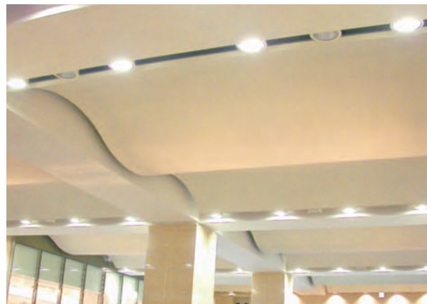
Ceiling : RIB 101 15mm (Curve Ceiling) Keihan Railway Kyobashi Station (Osaka Japan)
