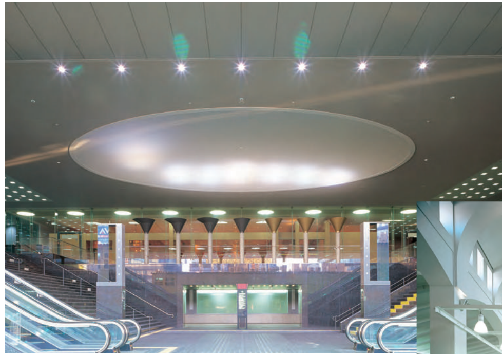
Ceiling : Travertine 12mm (Non-combustible Eaves Ceiling) Kyoto Station building (Kyoto Japan)
