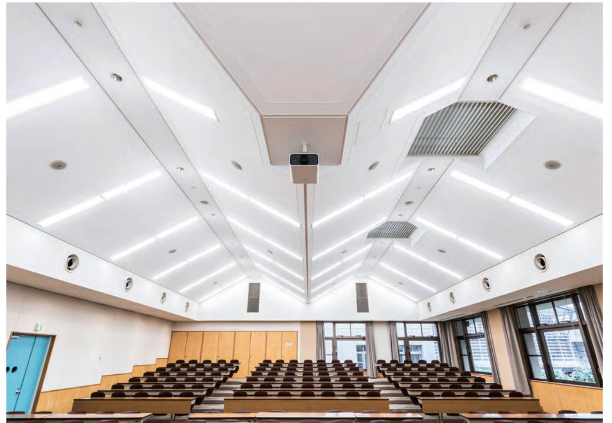
Ceiling : Travertine 9mm (Hybrid Ceiling) Meiji Gakuin University (Tokyo Japan)
