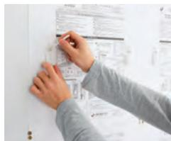
2. Line up the mounting hook with the pattern paper and affix it; hammer in the gypsum board nail; remove the pattern paper.
