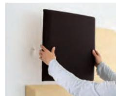
3. Mount panels from the bottom row upward until all panels are in place.
