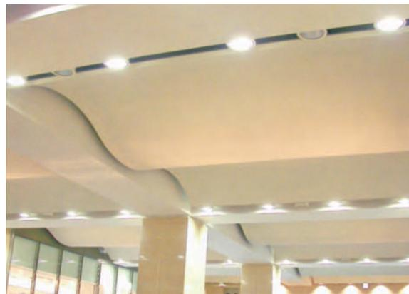
Ceiling : RIB 101 15mm (Curve Ceiling)
