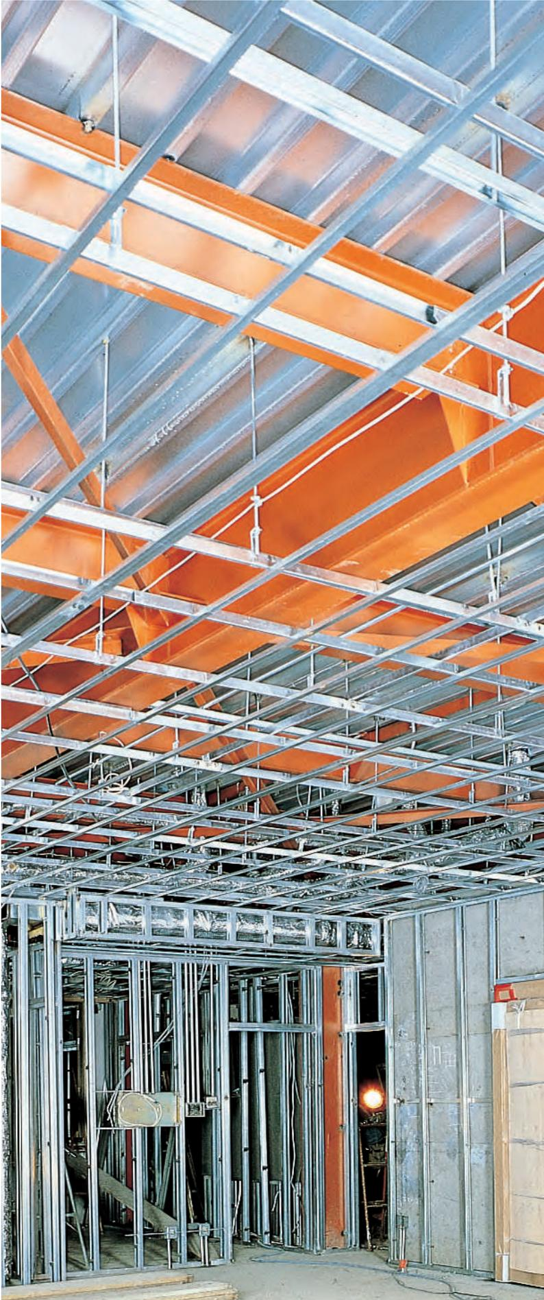
With a diverse lineup of functions, performance, size, and design, Daiken ceiling materials come with a selection of optimum Installation systems for each purpose. Including the most popular and economical Exposed T-BAR System, can be selected depending on the structure, ceiling construction, design concept, and budget. Easy maintenance also enables Daiken ceiling materials to offer longer ceiling life.
