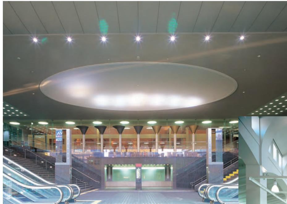
Ceiling : Travertine 12mm (Non-combustible Eaves Ceiling)
