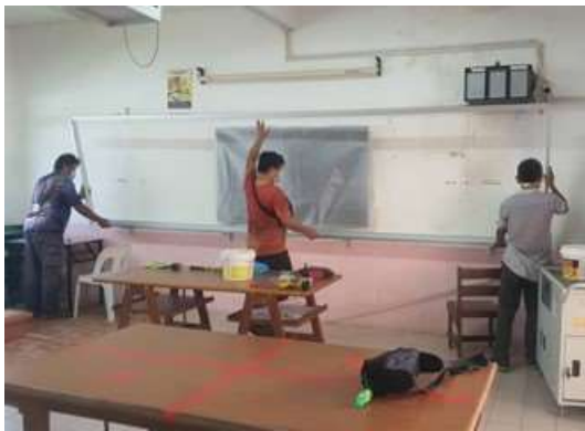
Photo 7: World Signcrafts was installing the whiteboard.
