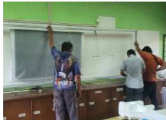
Photo 8: World Signcrafts was installing the whiteboard.
